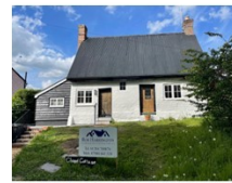
Period Restoration & Listed Buildings
